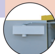
Self-closing door(s) with thermo-fuse
